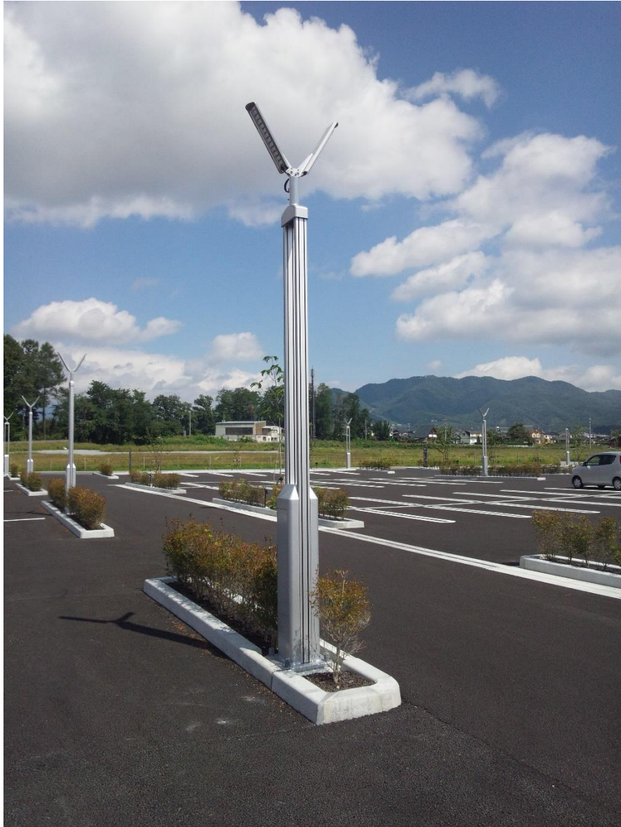
Fig. 2 Commercial power type LED light using commercial power supply
